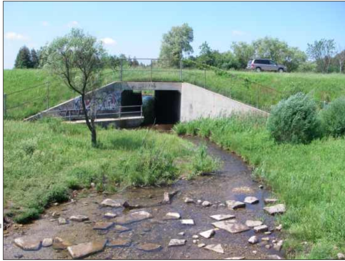
Hanlon Creek, looking downstream (west) toward the Highway 6 crossing.
