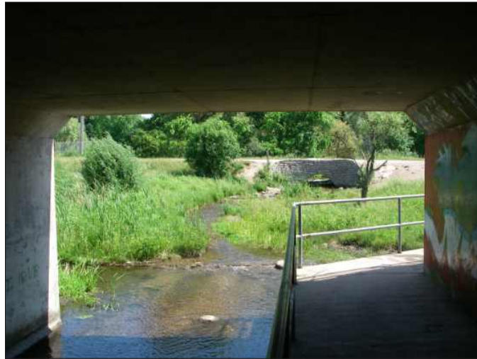
Hanlon Creek, looking upstream (east) from under the Highway 6 crossing.
